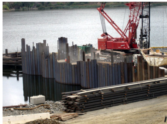
Construction of the closed cell cofferdam using PS 27.5 flat sheets.
