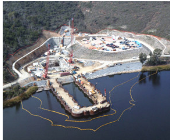
Aerial view of closed cell foundation for pump house inlet-outlet structure.
